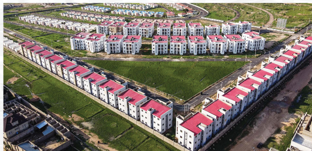
469 homes for low-income families at Family Homes Estate, Darmanawa Royal City, Kano State
